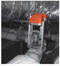
Globe valve retrofit with new UGVL linkage in Heinz Field, Pittsburgh, PA.
